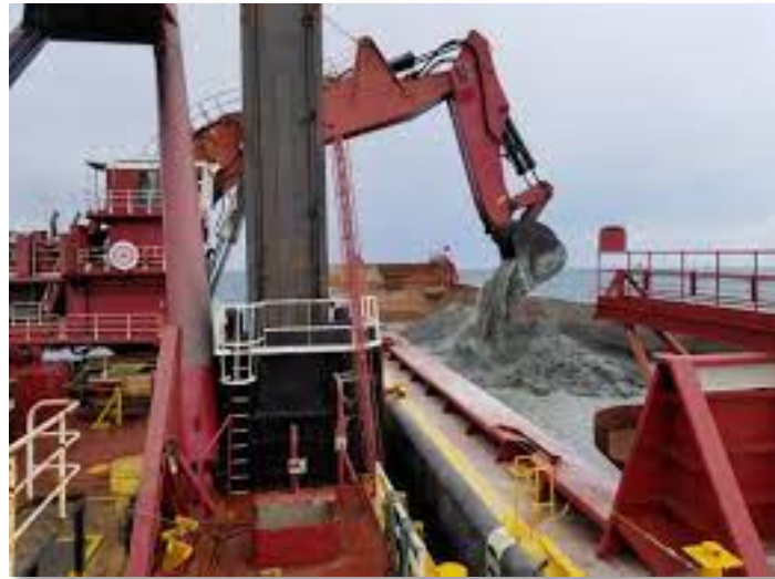
Hard Material Backhoe
